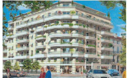
The exterior of 26 Blvd. Albert
